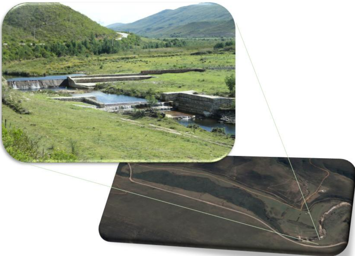
Figure 39: Gabion eastern border Upper Peatland Basin Source: Author's work
