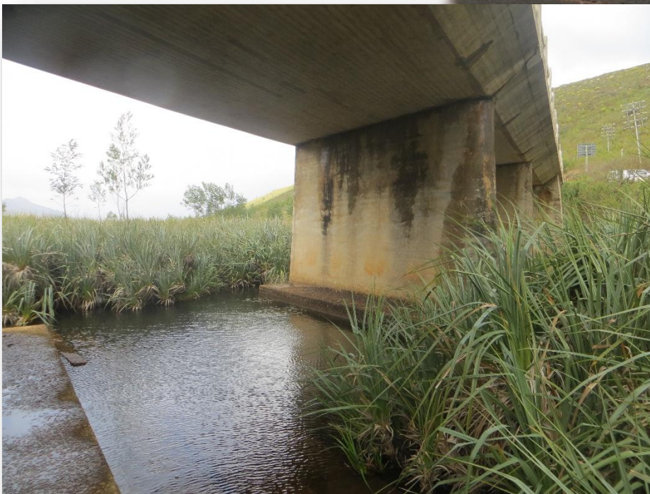
Figure 36: Bridge R62 Source: Author's work
