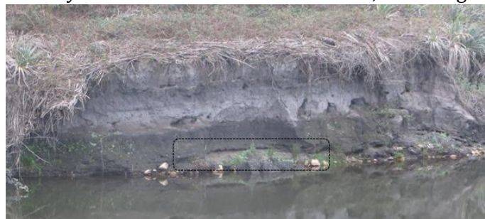
Figure 26: Piping Source: Author's work
