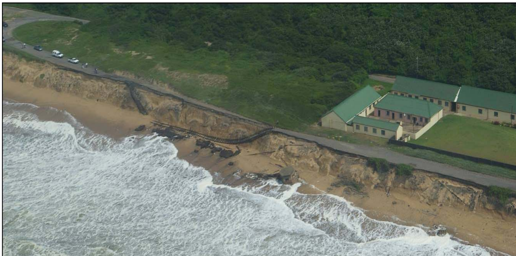
Figure 9: Damage to coastal roads cause by the KZN sea-level rise event of 2007 (Source A. A Mather)
