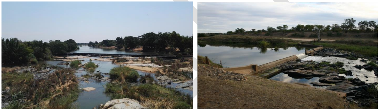
Figure 8 Mahale weir (left) and Letaba Ranch weir (right)
