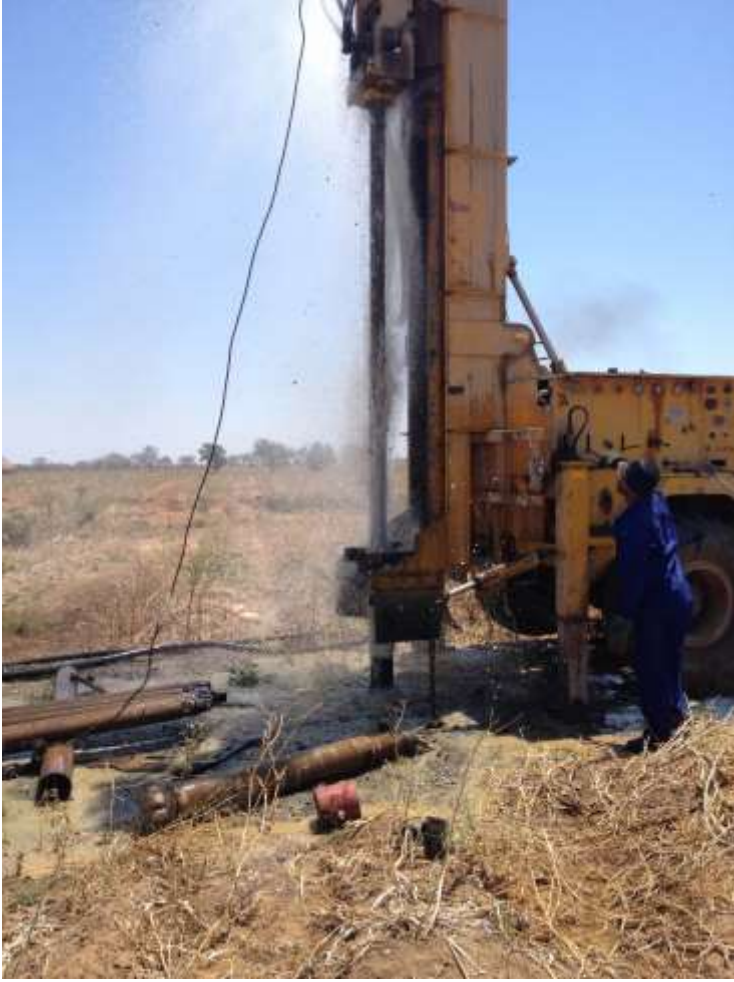
Figure III.2 example of the percussion drill during water strike
