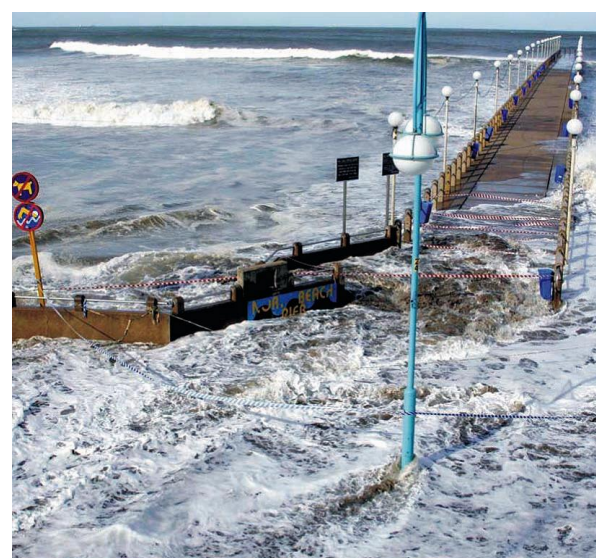
Damage from the March 2007 storm in KwaZulu Natal by high sea-levels and large waves; Top: Beach facilities on the lower South Coast; Middle: Flooding of George Hulett Place, Salt Rock; Bottom: Inundation of North Beach Pier, Durban
